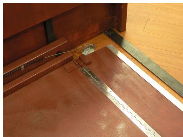
Fig. 15.2. Shown is the ramp with continuous hinge, return spring, cable, and cable housing.
